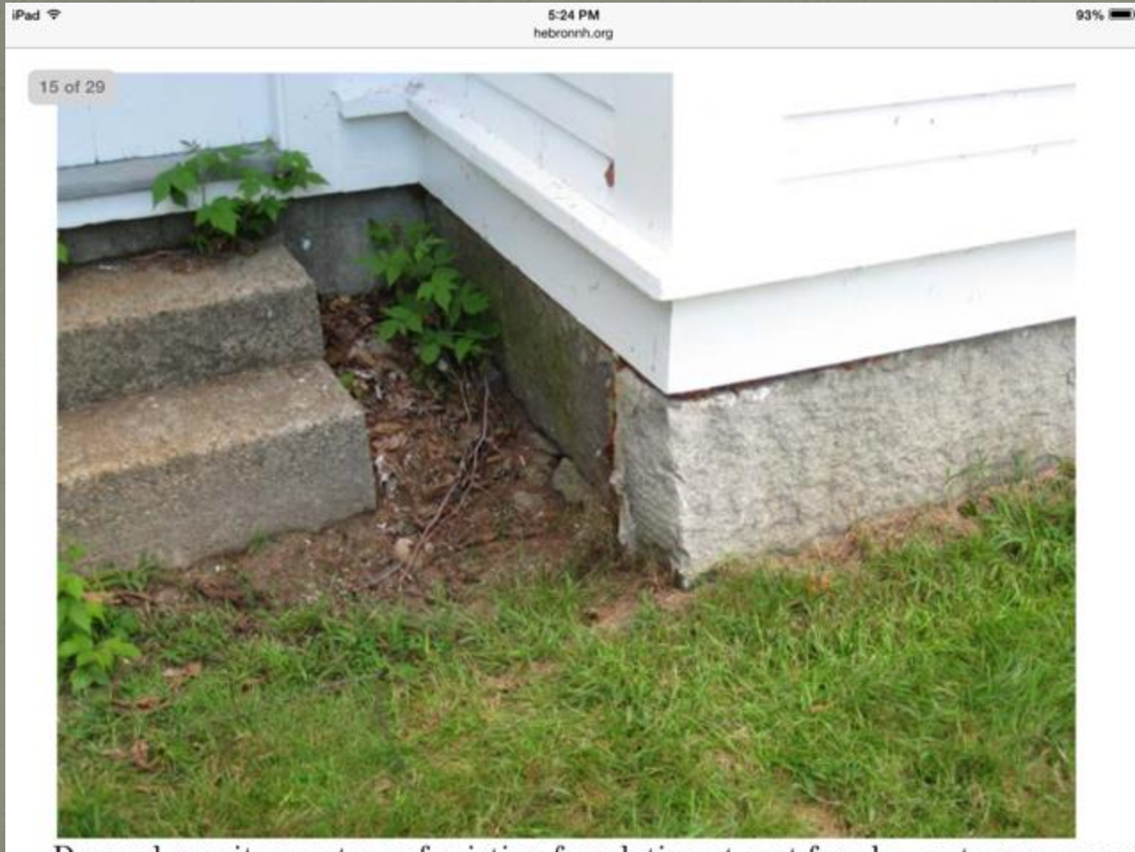
Dressed granite corners of existing foundation at east front, west rear corner.
