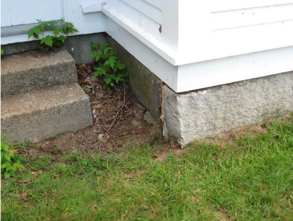
Dressed granite capstone of existing foundation at east facade – note gap caused by stone tipping outward.
