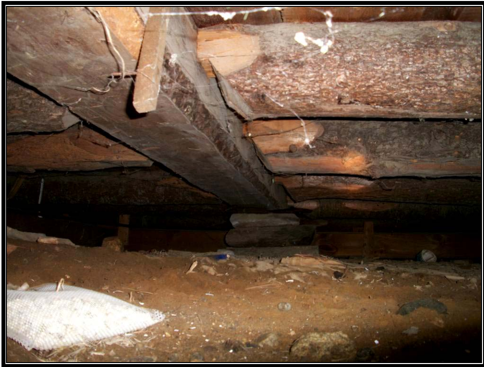
Photo 5: View of first floor built-up columns and notched floor joists.
