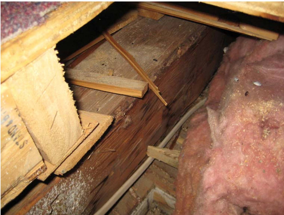
Original floor framing below Meeting Room has newer cross framing running perpendicular over the top. Note the split lath and plaster ceiling still attached to the bottom of the old timber joist. This is now hidden above the Selectmen's office by a poorly installed gypsum board ceiling.
