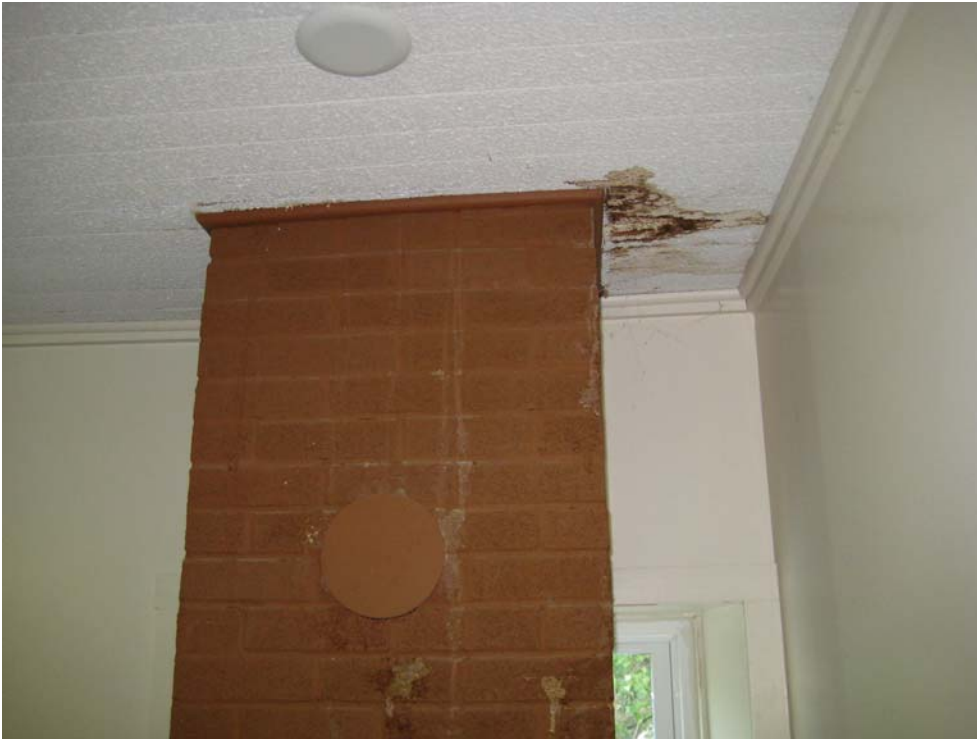
Water staining at chimney in Meeting Room is likely the result of flashing issues at the roof– note older wooden ceiling not original to building.
