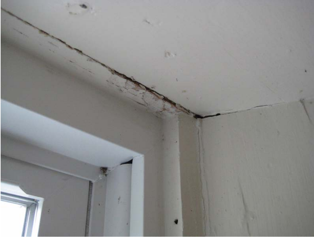
Typical water damage at windows in Entry Stairwell. Similar but less dramatic staining occurs in the Meeting Room windows
