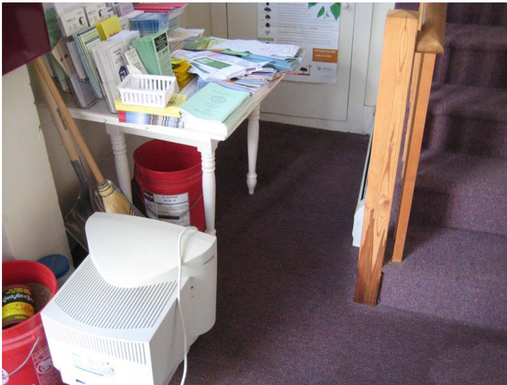
Water damage at bottom of stairs is likely caused by past or present leaking plumbing. Replace newel post (drawing dark staining materials up from bottom) if required.
