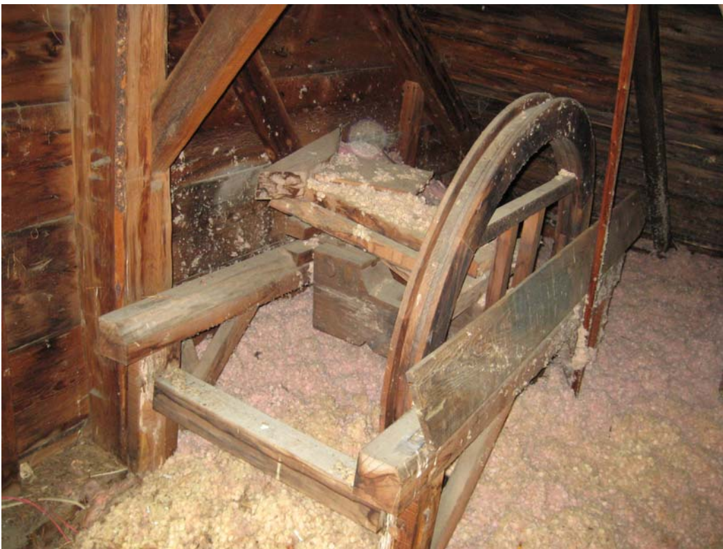
Northeast Tower northeast timber post and bell carriage for bell (previously removed to church across the common)
