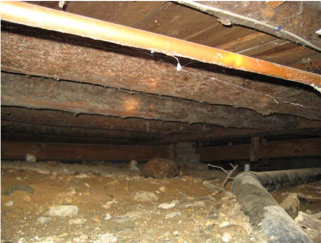
Existing crawl space with wooden plumbing chase and stone mid-beam support - note proximity of floor framing to soil and complete lack of insulation in floor system above.
