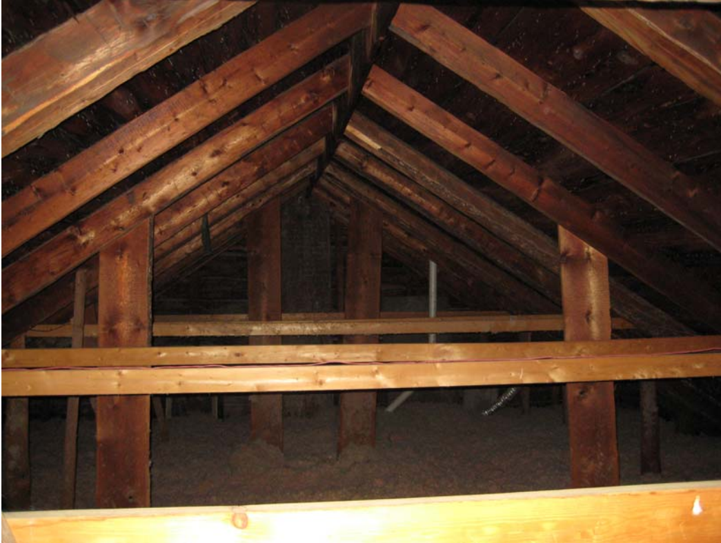
Attic with hand hewn and sawn common rafters
