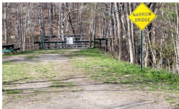
Access bridge over the Cockermouth River
